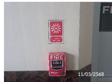
Fire Alarm Manual Station
