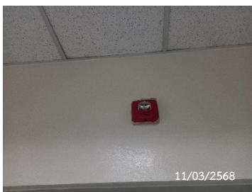
Indoor Selectable Output Speaker
