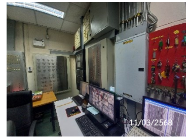
Graphic Annunciator Fire Alarm System
